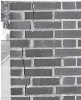
A large crack runs through the bricks at the Middle School. This can be seen from the rear driveway approaching 20A.
