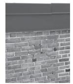
Cracks are visible on the kitchen side of the Cafeteria wall at Windom Elementary.
